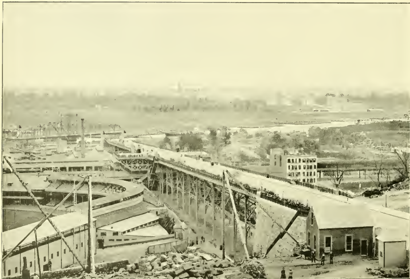
VIADUCT AND HARLEM RIVER, FROM NEW SPEEDWAY -- One Hundred and Fifty-fifth Street.
